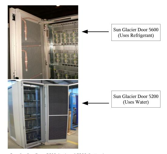
Figure: Sun Cooling Door 5600 (top) and 5200 (bottom)
